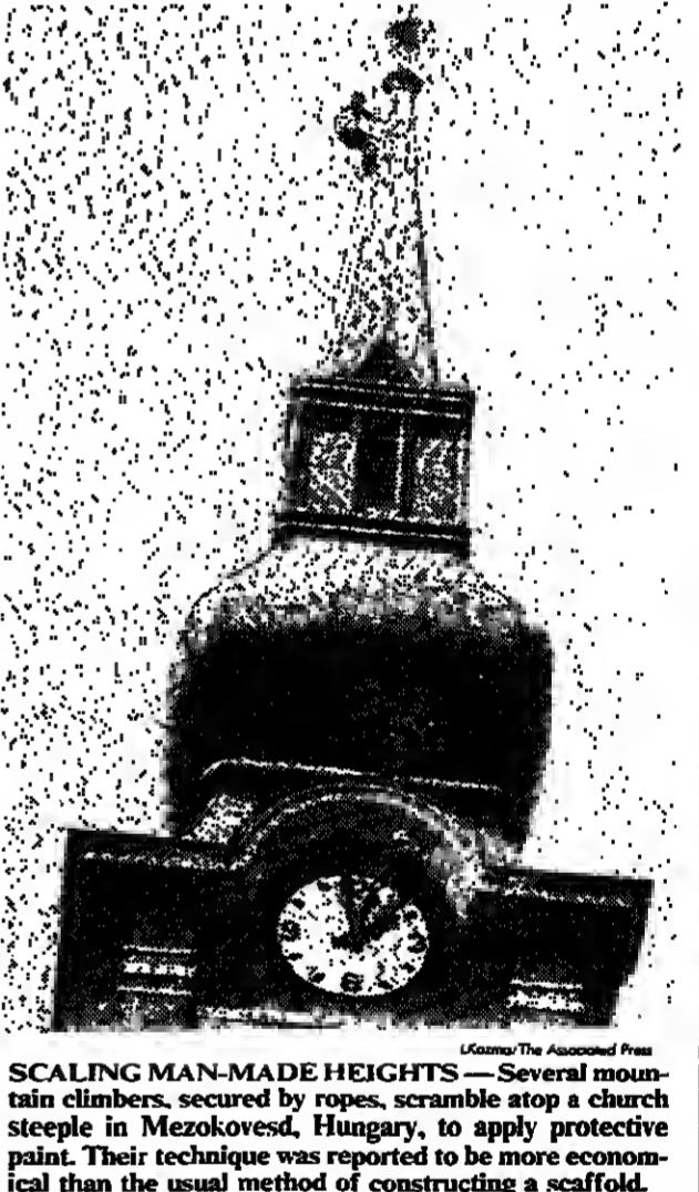
SCALING MAN-MADE HEIGHTS — Several mountain climbers, secured by ropes, scramble atop a church steeple in Mezokovesd, Hungary, to apply protective paint. Their technique was reported to be more economical than the usual method of constructing a scaffold.
